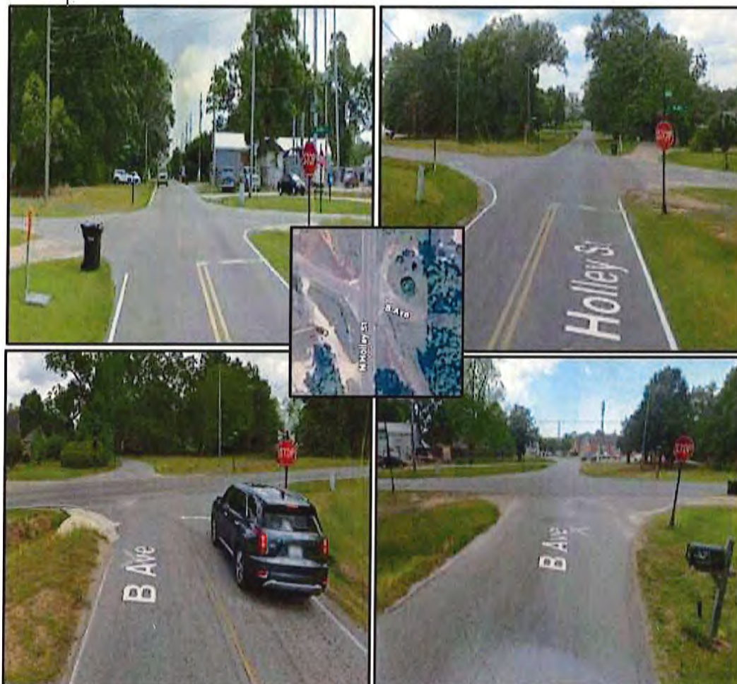
Figure 2.5 Intersection B Avenue/ N. Holley Street Images
